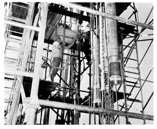
D. B. LIST (7123), assistant project engineer for Sandia's earth motion instrumentation, checks the four canisters prior to lowering them into the hole. When at proper depth, motors inside the canisters precisely positioned the internal seismic and accelerometer instruments directly in line with the nuclear device.
